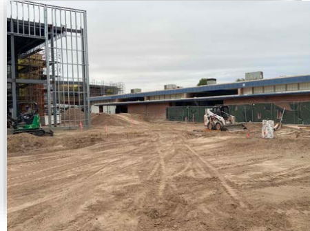
Figure #14 – Relocate Excavated Dirt From Trench December 17, 2020
