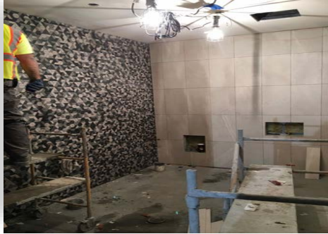
Figure #19 – Install Tile in Restroom 1D12 December 23, 2020
