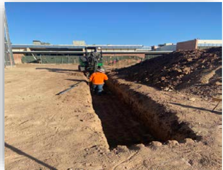
Figure #10 – Excavate Amphitheater Foundation December 14, 2020
