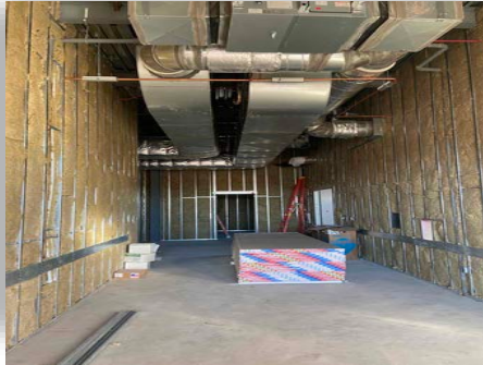
Figure #13 – 2 nd Floor North Grid Insulation December 16, 2020
