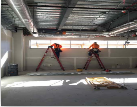
Figure #1 – Building & Installing Window Frames December 1, 2020
