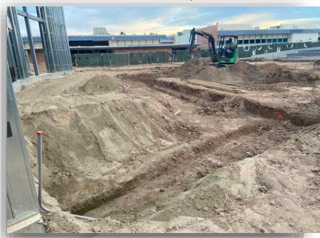
Figure #18 – Excavation of Amphitheater Foundation December 22, 2020
