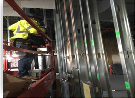
Figure #20 – Vent, Water, Gas, & Condensate in Labs December 28, 2020
