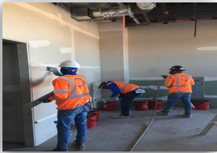
Figure #15 – Cut, Fill, and String Tape 1 st Floor December 18, 2020
