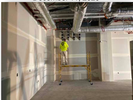
Figure #11 – Cut, Fill, and String Tape December 15, 2020
