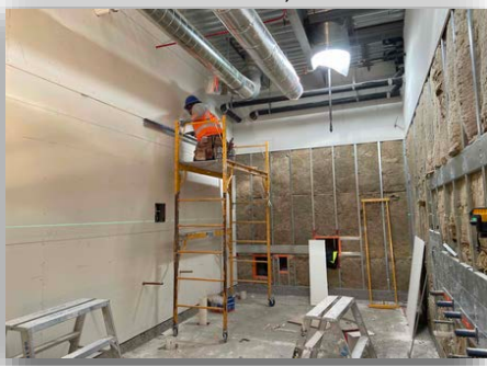
Figure #17 – Installing Drywall on 2 nd Floor Restrooms December 21, 2020
