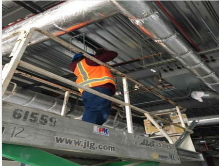
Figure #7 – OH Refrigerant Piping @ Second Floor December 9, 2020
