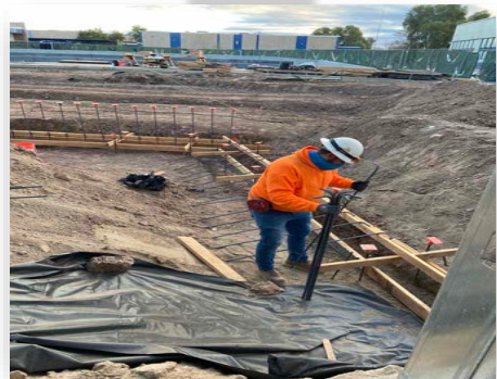
Figure #22 – Installing Rebar Around Footings December 29, 2020
