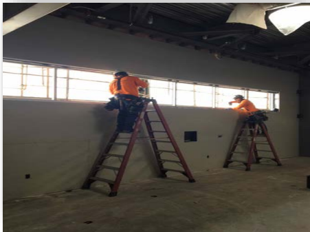
Figure #9 – Install Window Frame 2nd Floor Classroom December 11, 2020
