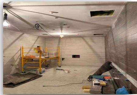
Figure #16 – Tile Installation, 1 st Floor Restrooms December 18, 2020
