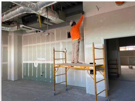
Figure #21 – Interior Taping on 1 st Floor Multiple Rooms December 28, 2020
